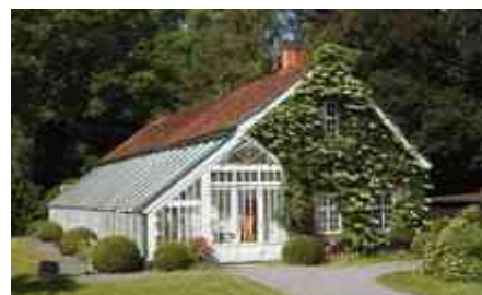
Orangerie in Hasses Park | Foto: Torsten Krüger, Bremen
