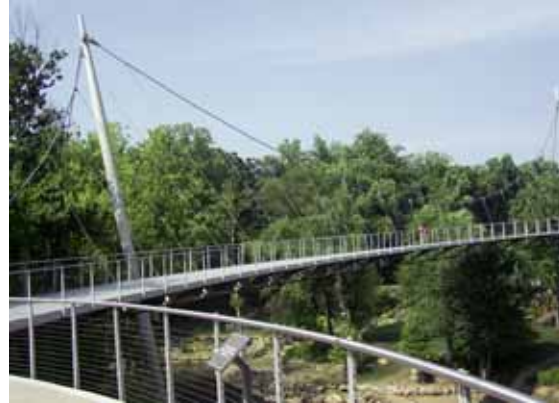
The new Liberty Bridge enables a view of the waterfall and serves as a symbol of Greenville's prosperity.
